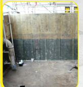
A full concrete repair and protection system solution was developed with Thelwell Flooring: All of the damaged concrete was removed mechanically followed by blastcleaning of all surfaces; the damage was repaired and made good with polymer modified concrete and mortars from NCC and allowed to cure; finally the surfaces were all coated with Atako ATB-300 GL, a highly acid and chemically resistant, vinyl ester based, glass fibre reinforced concrete protection system.
